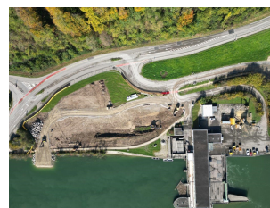
Construction of the new fish pass at the Flumenthal hydropower plant.
